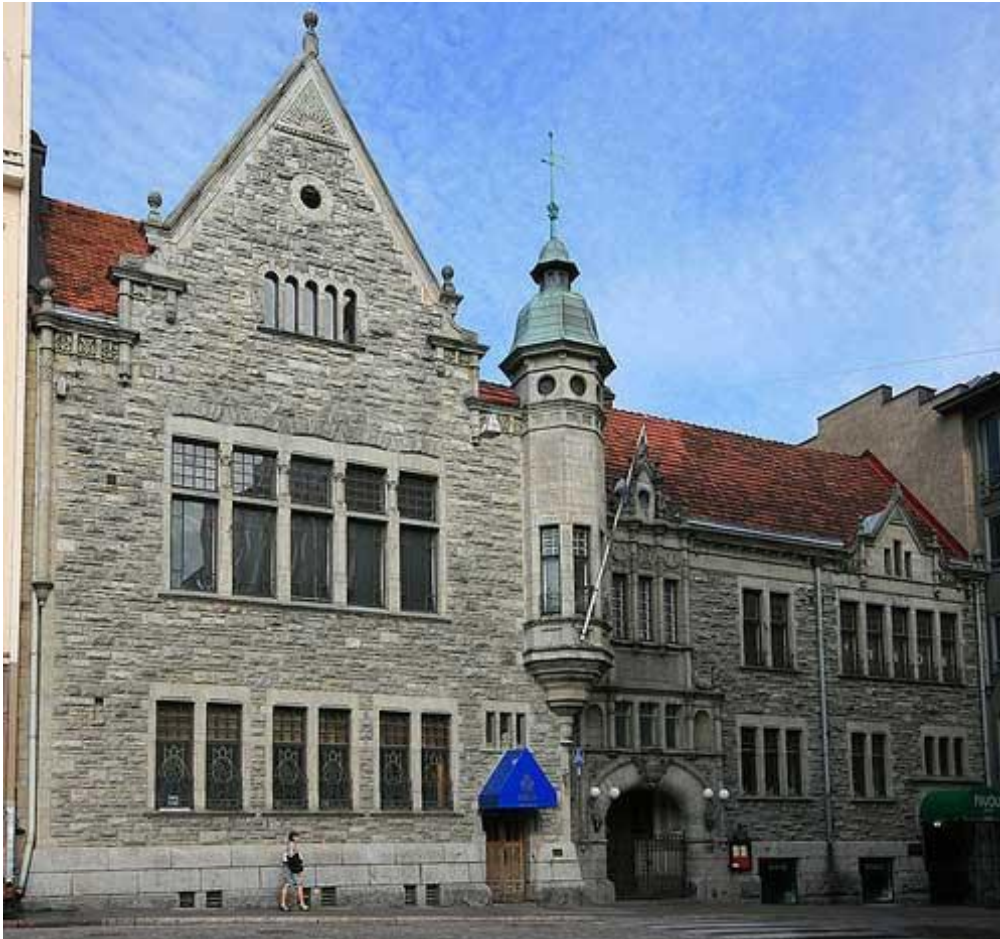
Nyland Nation house through the gate you go to the Rivoli hotel behind this building.
