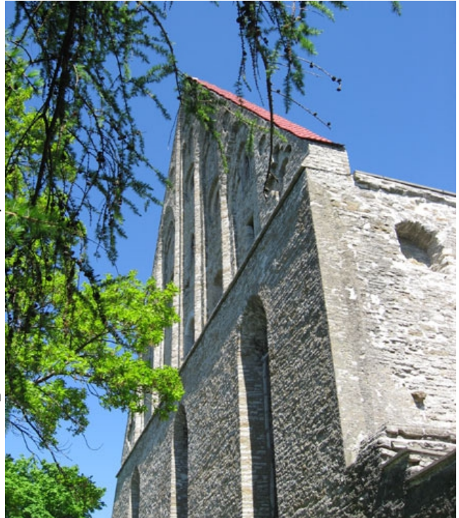
Front of the church (west)
